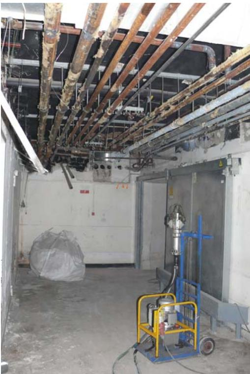
The environment-friendly, hydraulic DARDA system – Combi-Shears and electric power unit - cleared out 10,000 meters of metal pipe.
