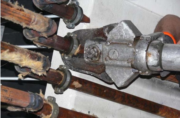
Using the easy-to-handle Combi-Shears HCS6, a single person can quickly cut through metal pipes noise- and odor-free.
