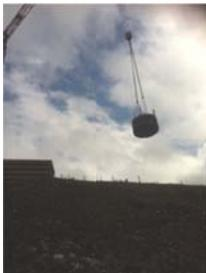
A crane is used to lift off the hydraulically split pile heads and remove them.
