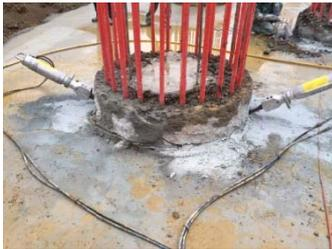
A combination of 2 DARDA splitting cylinders quickly break up a reinforced pile head in a controlled and user-friendly manner.
